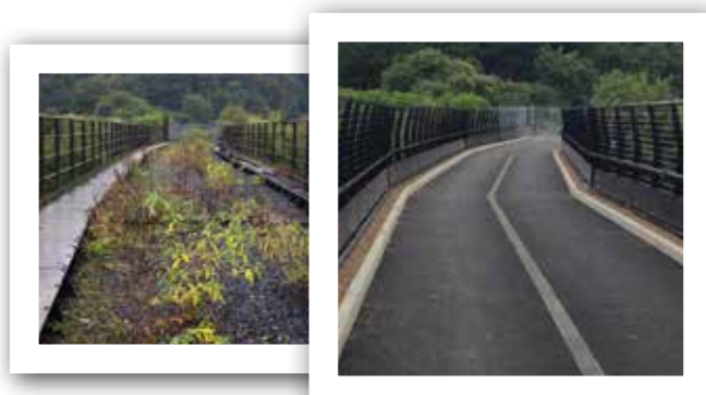
Cart Road 52 – Before and after
