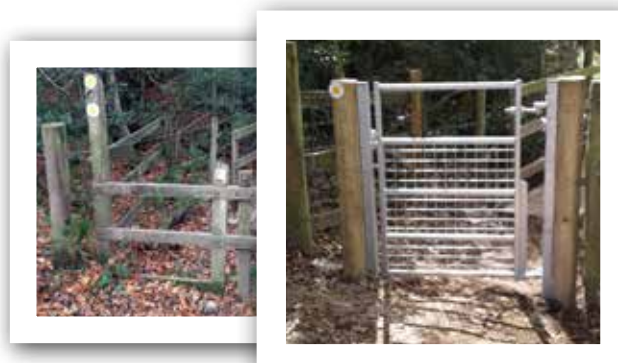
Radyr 27 – broken stile replaced by gate
